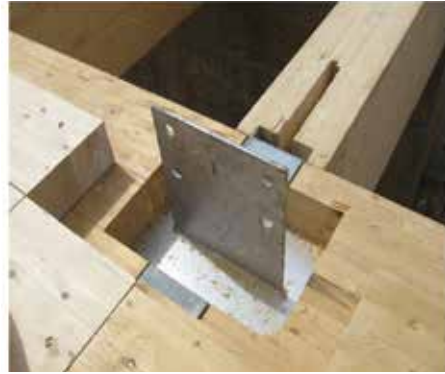
Modern Computer Numerically Controlled (CNC) connections provide the ability to fabricate joints with precision. This is especially useful when fabricating joints on large members with complex shapes.
