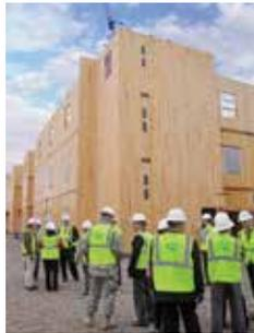
Made from CLT, the four-story Candlewood Suites Hotel at Redstone Arsenal, Alabama, had to meet Anti-Terrorism and Force Protection standards required for every structure built on a U.S. military base. Extensive engineering analysis was used to determine compliance with blast-resistance criteria. Photo credit: Lend Lease
