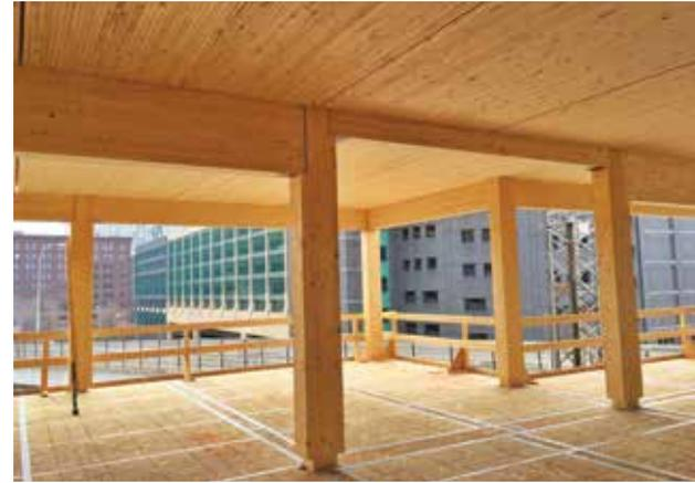
Designed by MGA, the seven-story T3 building in Minneapolis includes glulam columns and beams, and NLT floors.
