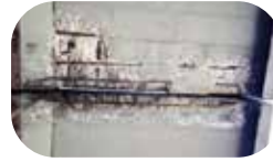
CONCRETE SPALLS
