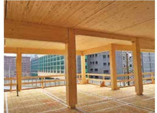
Designed by MGA, the seven-story T3 building in Minneapolis, Minnesota, includes glulam columns and beams, and NLT floors. Photo courtesy of StructureCraft
